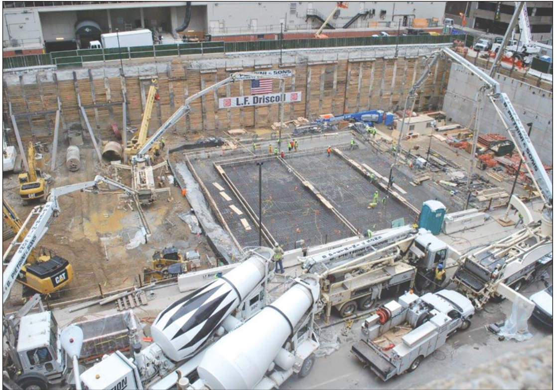
The concrete pour consisted of 3,800 cu. yds. (2,905 cu m) of concrete.
