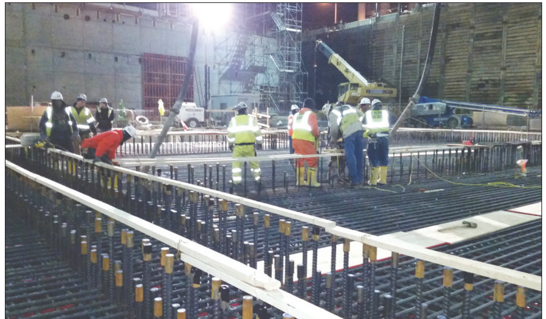
Approximately 400 tons (362.8 t) of reinforcing steel was placed.
