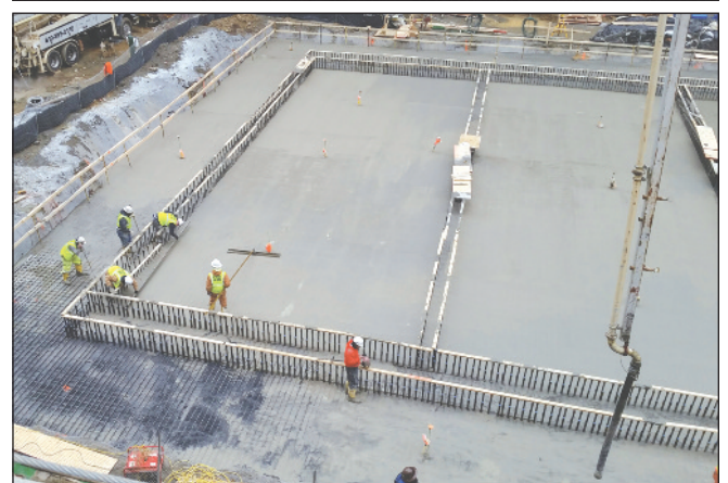
A crew of approximately 45 people pumped, placed and finished, and also coordinated trucks to the various concrete pumps.
