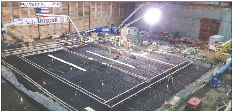
Concrete began discharging at approximately 1:45 a.m. into a Schwing 47SX and 39SX pump that poured directly in the foundation from Arch Street.
