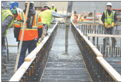
The continuous flow was required so that no wet concrete went over hardened concrete.
