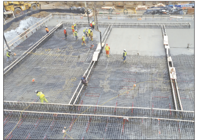
The concrete pour consisted of 3,800 cu. yds. (2,905 cu m) of concrete.
